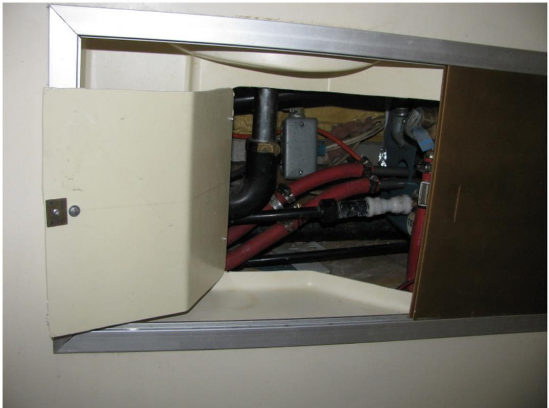
Showing the “T’s”, the ball valve, and the check valve that now blends some cold water into the hot water going to the bathroom sink. The valve handle is just off straight vertical where it would be completely shut – this position lowers the hot water coming out of the faucet to a comfortable 110 degrees from the approximately 180 – 190 degrees in the tank.
